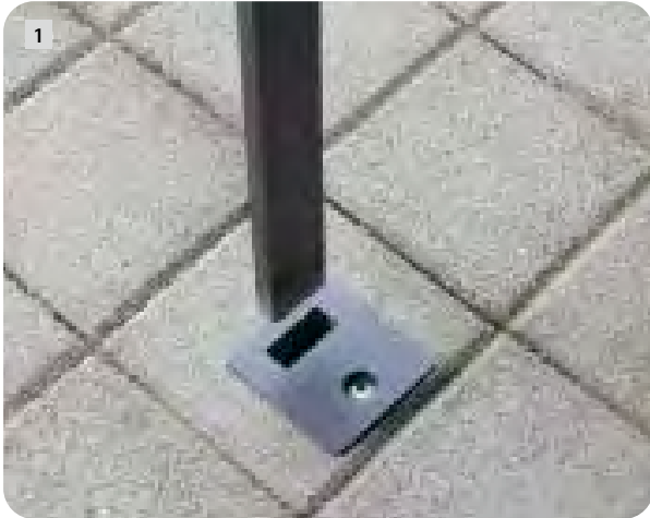
1 Insertion of the bicycle-stand in the ground sleeve...
