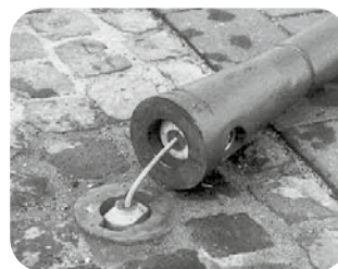
3 | Bollard system after damage
